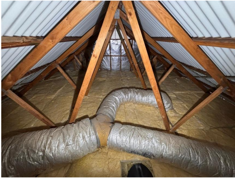
Figure 7: image of the insulation upgrade in the roof with R3 roof batts laid over existing material. CosyWrap also sealed any holes in the ductwork of the AC to make it run more efficiently. CosyWrap were in attendance to talk to all attendees about the insulation and draught sealing work they could do – and were inundated with conversations.
