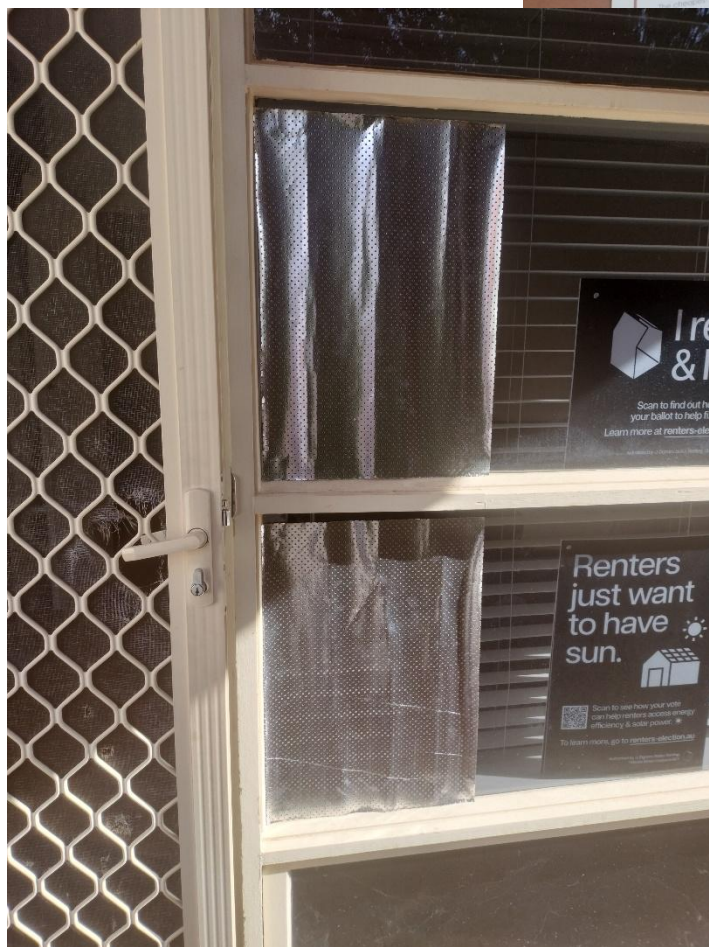
Figure 4: A display of Renshade - a perforated reflective film used to reflect direct sun light. It was downstairs as we didn't allow people upstairs. The front door also had EVM Slimline tape installed to block draughts.
