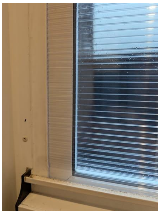
Figure 124: People have recently started using clear corflute sheets to mimic double glazing. This image shows it cut to fit against the glass with the channel laying horizontally. This will insulate the window, losing less heat to outside in winter. You can also use bubble wrap to insulate glass or lower your outdoor roller shutters to mimic double glazing and keep the heat in in winter.
