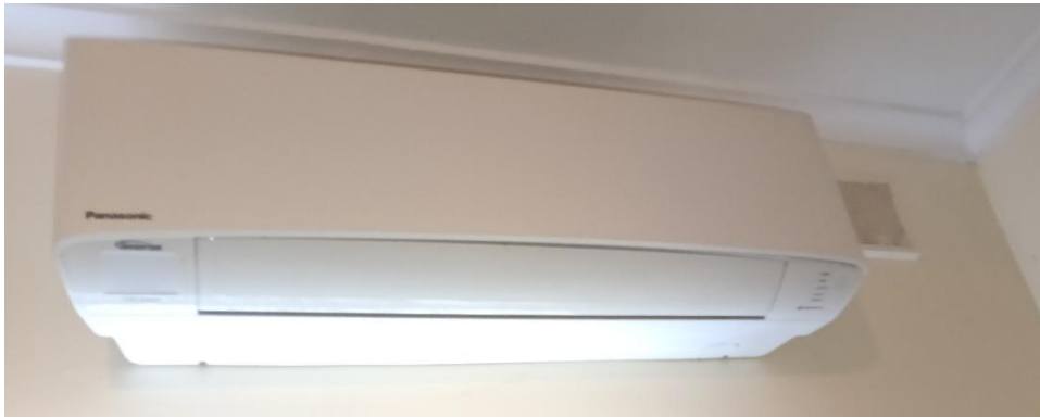
Figure 135: a small wall mounted reverse cycle air conditioner is the most efficient heater. Large and ducted systems can cost more to run. If you buy a new AC, get the highest star rating that you can afford. Check the running costs here at the Energy Rating website .
