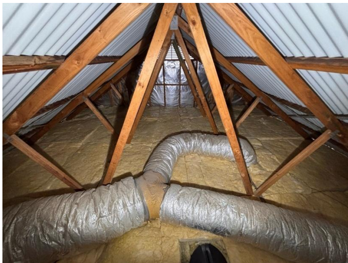
Figure 157: The SHD house had its insulation tidied up, and extra layer laid over top. This is what it looked like afterwards - a consistent even layer with no gaps. Work completed by Cosywrap .
