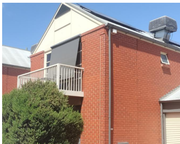
Figure 8: where possible, this house with no eaves to shade windows or walls, was able to use external shading to reduce the heat build-up via windows facing north. They have a cafe blind and bushy shrubs.
