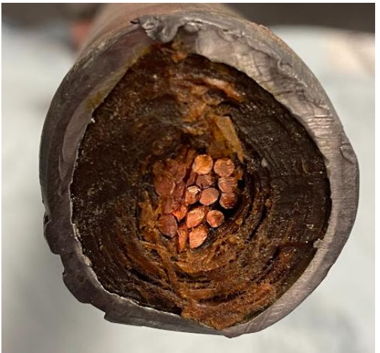
11kV paper insulated lead covered Cables 1960's & 1970's
