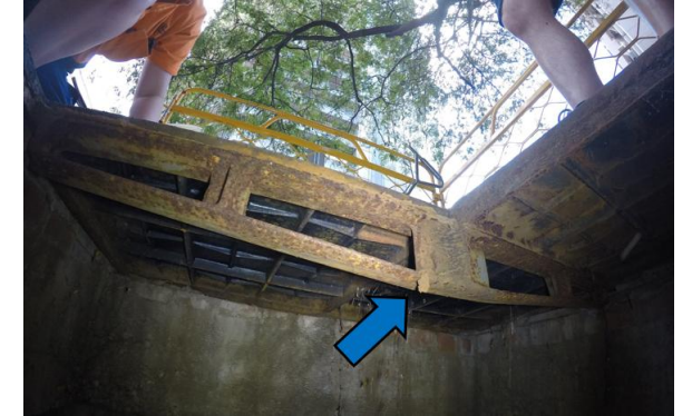
Collapsing lid support
